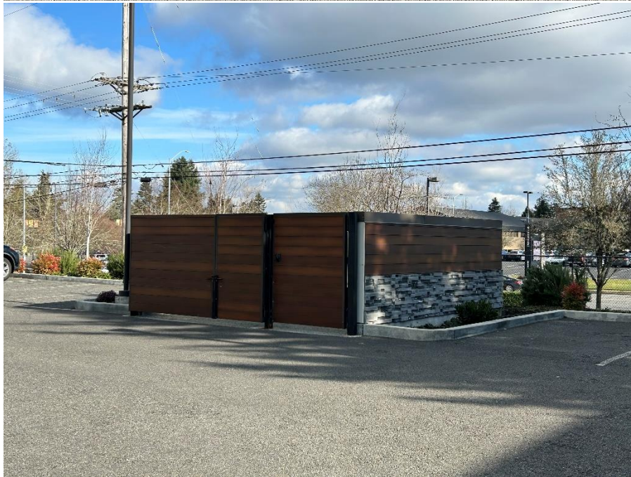
Gated enclosure for frontload collection container
