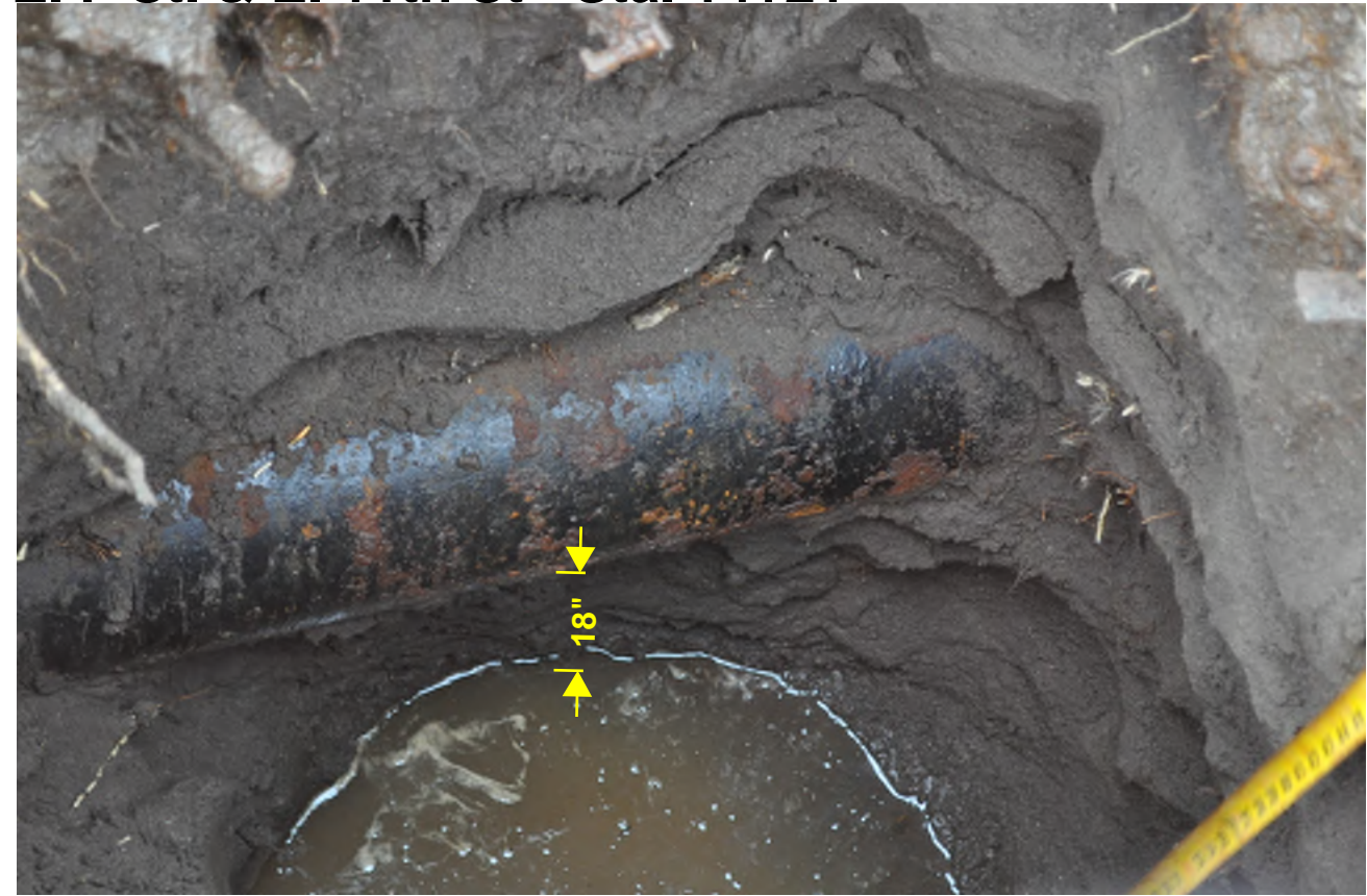
*Bottom of pipe to top of water-18"
