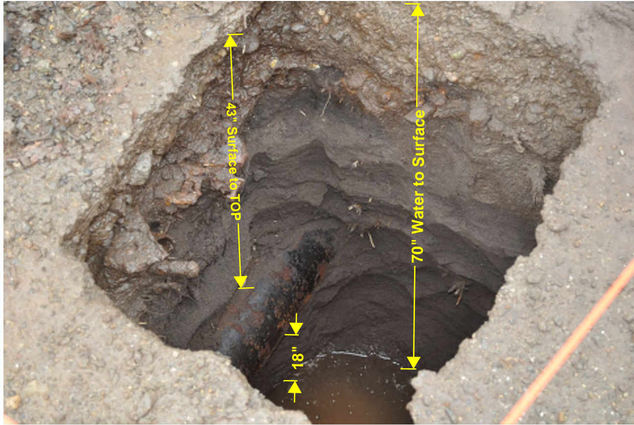
*Bottom of pipe to top of water-18"
