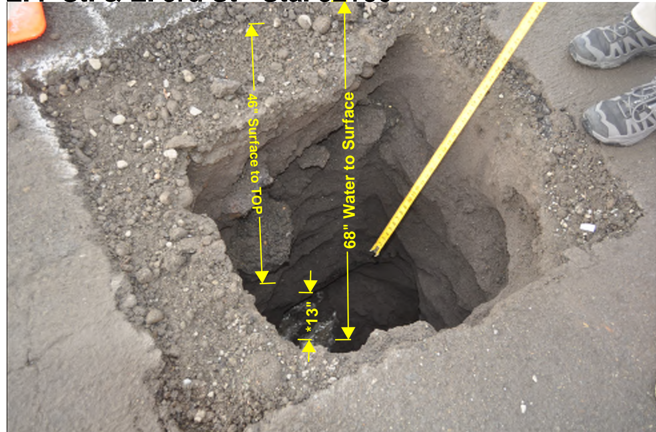
*Bottom of pipe to top of water-13"
